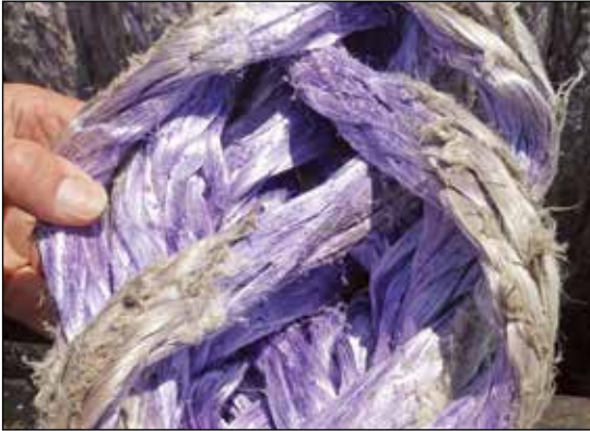
Inspection of hollow core area of 12x12 Strand rope. In picture above, no internal wear is observed. Exterior yarn abrasion is noted as 'light' and not a problem.
